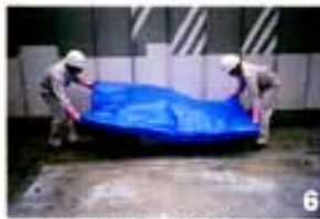
Covering with a plastic sheet
