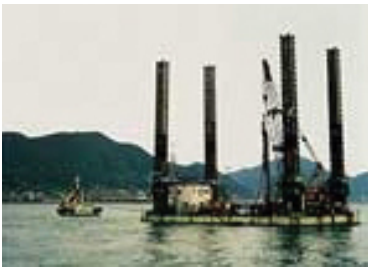
Demolition under Water
