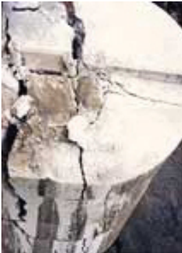
Demolition of Pier
