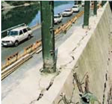
Demolition of Retaining Wall
