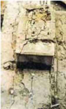
Demolition of Concrete Foundation for machinery
