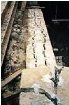
Demolition of Temporary Concrete Structure
