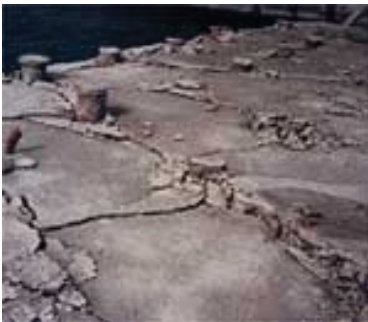
Demolition of Pier
