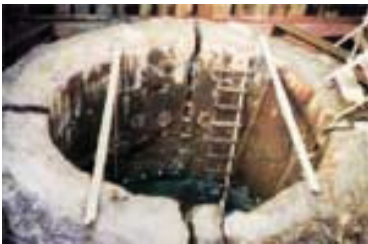
Demolition of Pillar
