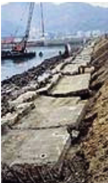
Demolition of Retaining Wall
